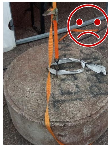
The S hook will come loose as wind moves the structure. The fastening is not locked to the mounting point.
