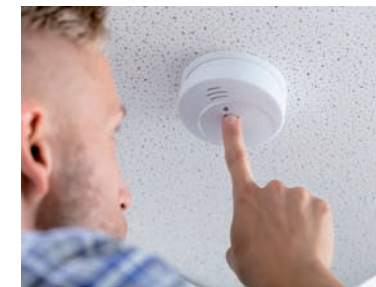
The resident is responsible for testing the smoke alarm once a month.
